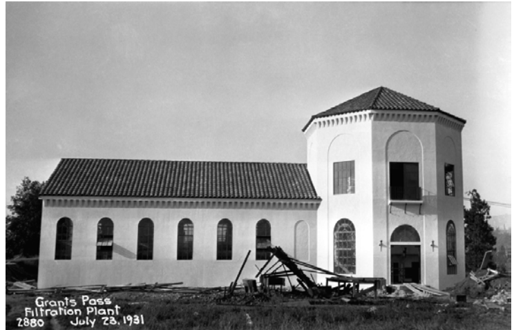
Filtration Plant Constructed July, 1931
