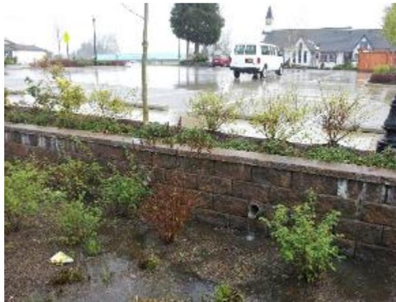
*Figure 3-4. Pervious concrete and a stormwater planter were chosen for this public Park and Ride parking lot in Veneta, OR.*
