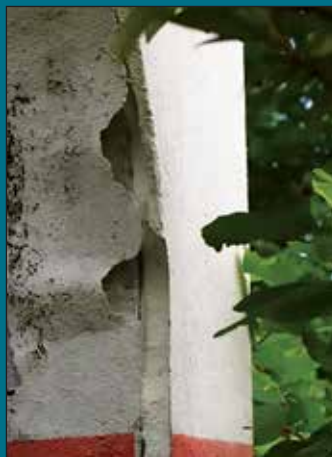
Photos show delamination and loss of integrity of walls and water bearing structures and roof patches.
