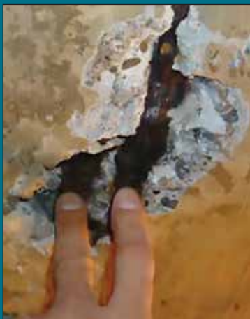
Photos show delamination and loss of integrity of walls and water bearing structures and roof patches.
